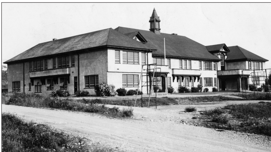
North Vancouver High School, 1938. Source: North Vancouver Museum & Archives, #5339
